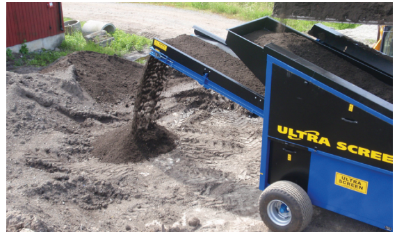
Screening soil at 15mm at rates of 45 tonnes per hour
